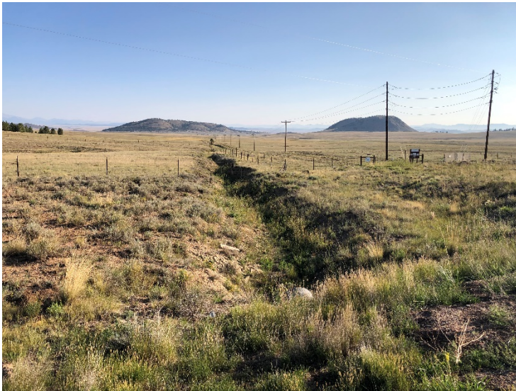
Photo 1. Avoidance Area 1, looking northeast from US 24 ROW. Large stormwater drainage feature that drains to the north (into the background), but the origin and source is unknown.
